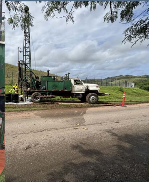
Drilling Rig Setup
