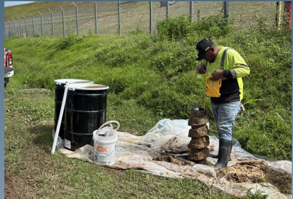
Checking depth of installed materials
