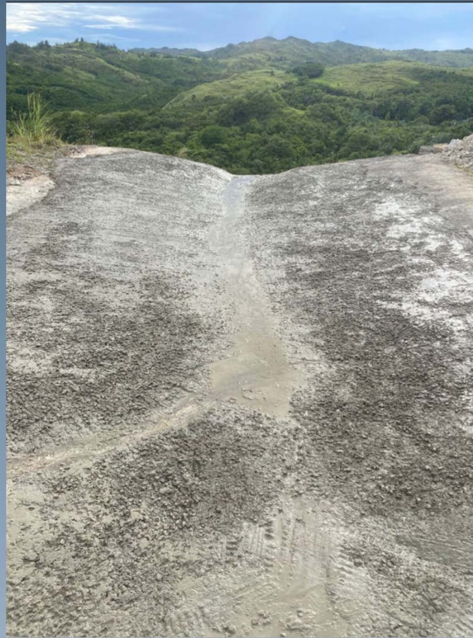
Storm Swale Repair Construction (location 45)
