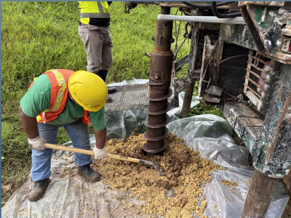
Borehole Drilling
